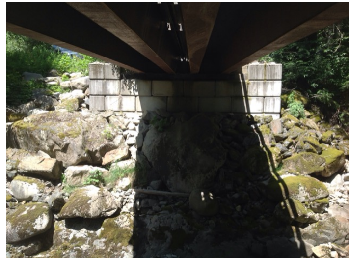
Right Bank Abutment when facing downstream
