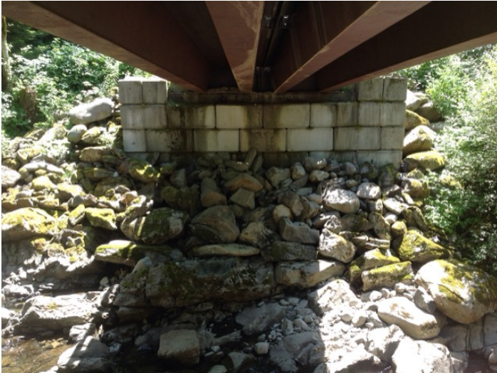
Left Bank Abutment when facing downstream
